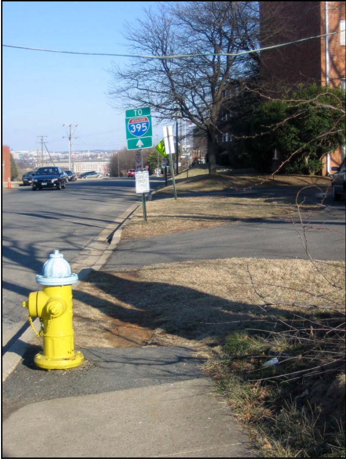
Missing sidewalk on Southgate Road between Ode and Orme Streets
