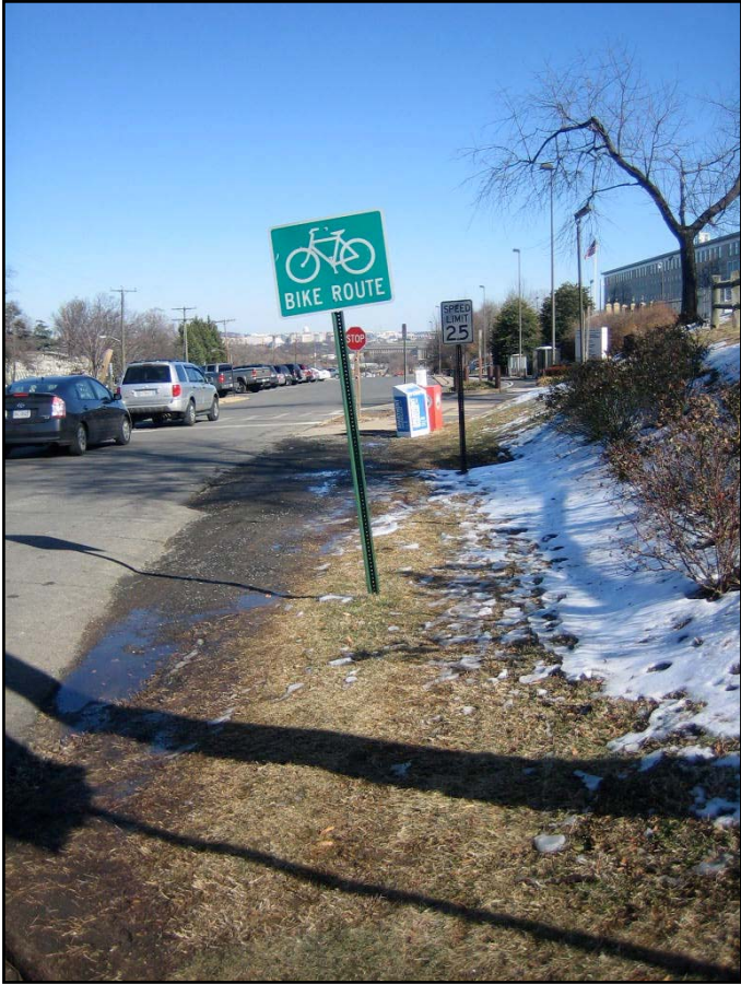
Missing sidewalk at bottom of hill abutting Foxcroft Heights Park
