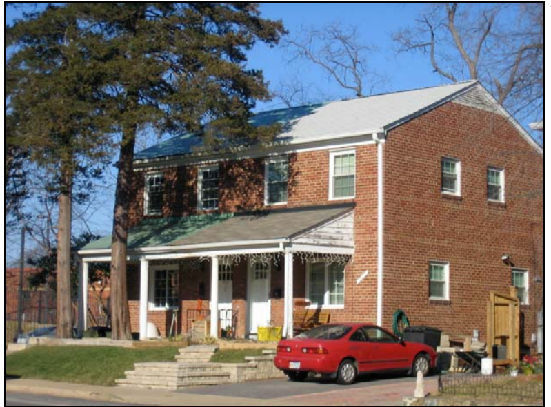
Duplex dwelling on Orme Street
