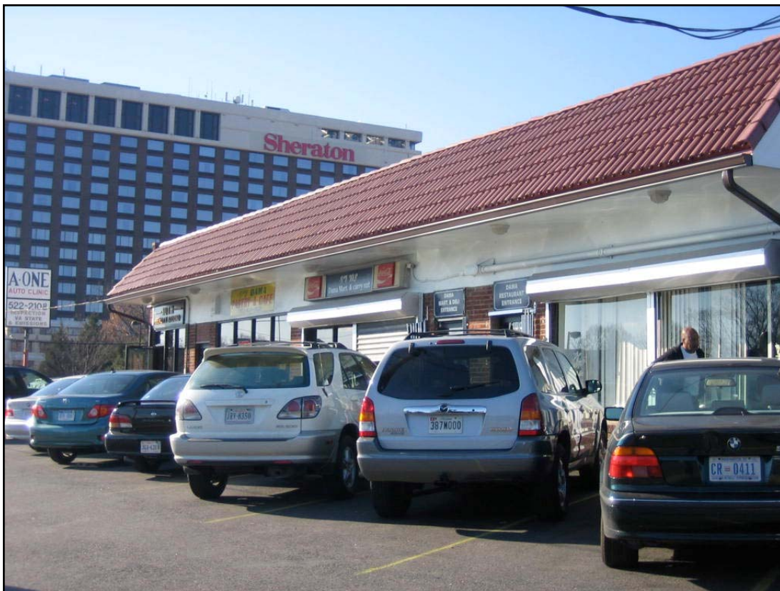
The Dama restaurant and café that comprises that main part of the Foxcroft Heights commercial strip
