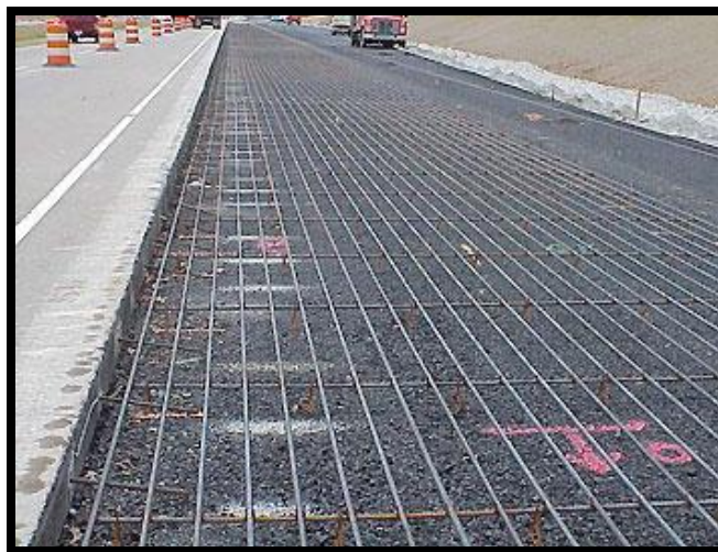
11: A modern example of steel rebar in CRCP.
