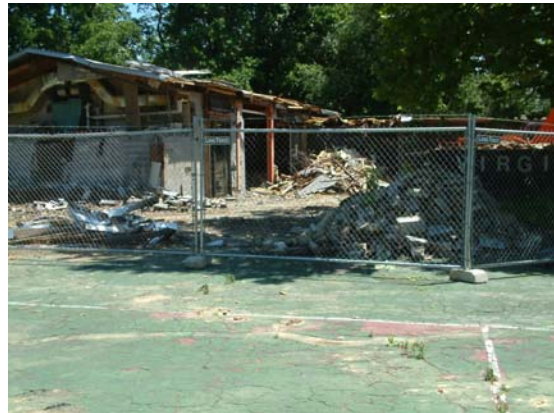
The Walter Reed Rec Center being demolished (2004).
